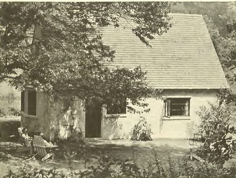
Familiar to readers of Woman's Home Companion is the "Home Keeping House" at Westport, Conn. Random sized concrete masonry forms its walls. Estimated cost is $2,500. Frank Harper Bissel, architect, New York City.
